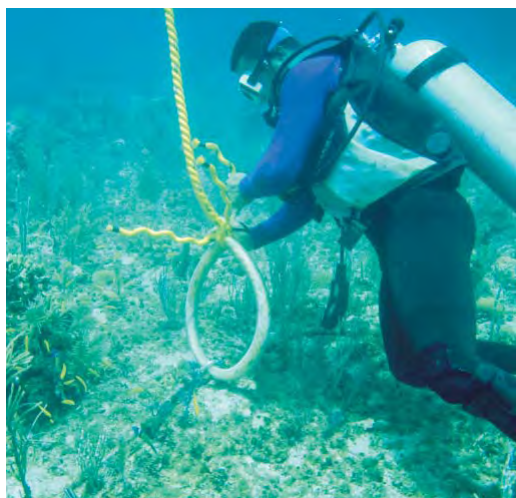
A diver installing a mooring buoy to protect a reef from anchor damage
