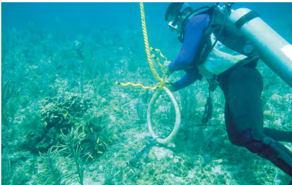
A diver installs a mooring buoy to protect a reef from anchor damage.
